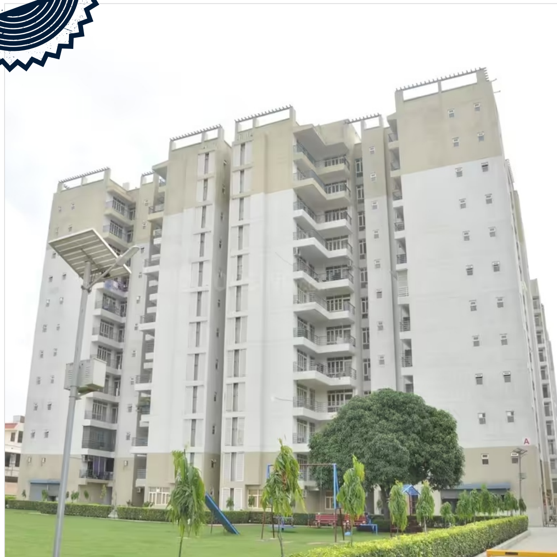
21 st MILESTONE RESIDENCY Raj Nagar, Ghaziabad
